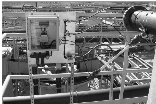
*Illustration 1: Turbulent Flow Sampler
